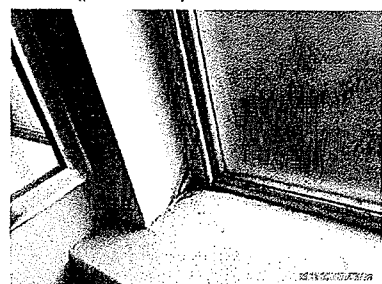
Bathroom: Windows/screens/window safety devices (photo 5 of 5)
