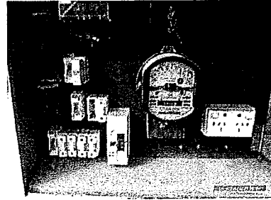
Security/Safety/Utilities: Electricity Meter (photo 2 of 3)
