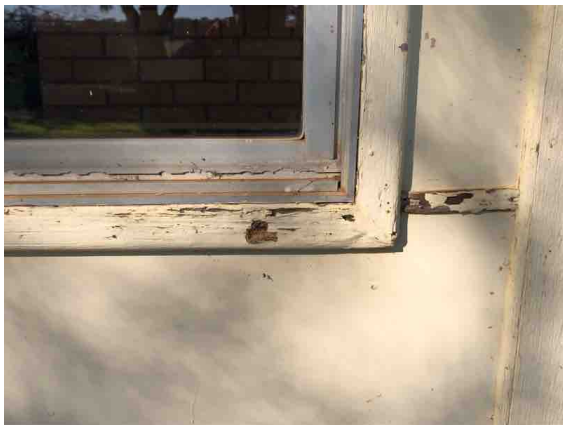
The deteriorating paintwork.
