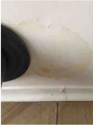
The ceiling is water stained around the fire flue.
