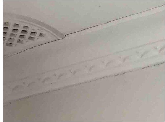
The cournice is cracked around the fire flue.
