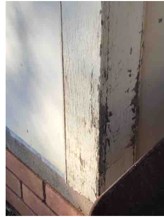
The deteriorating paintwork.
