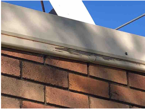
The deteriorating paintwork.
