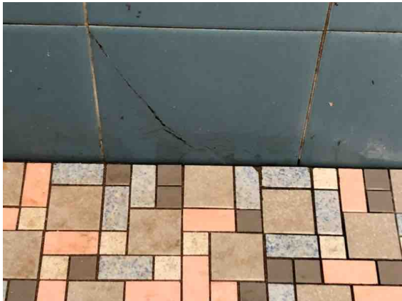
The cracked wall tiles in the shower area.
