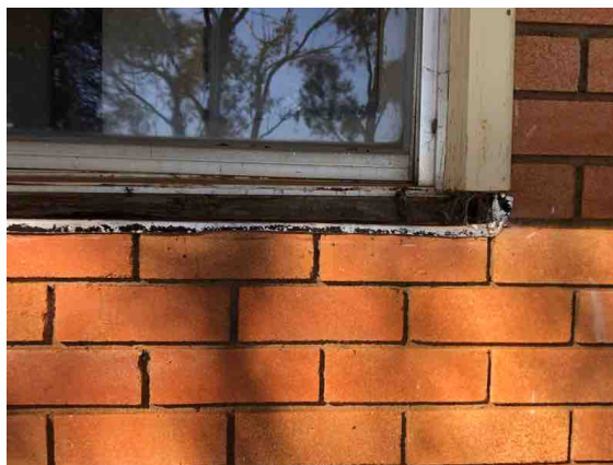
The timber window sill is damaged and needs repairing.
