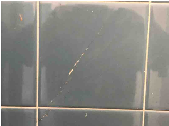
Cracked wall tiles in the shower area.
