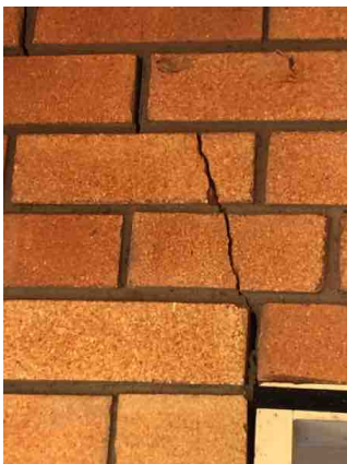
Vertical cracking.
