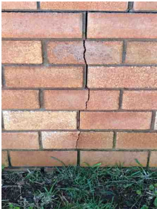
Vertical cracking
