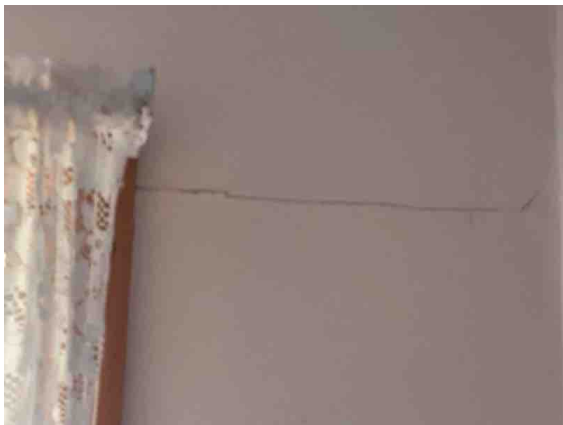
Wall cracking.
