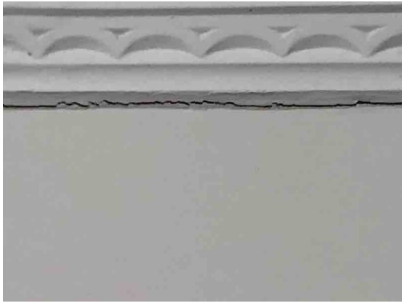
The cracking cornice.
