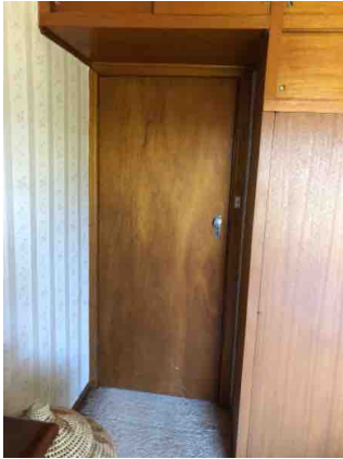
The entry door to the bedroom needs easing.
