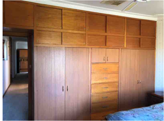
The wardrobe doors are binding and need easing and adjusting.
