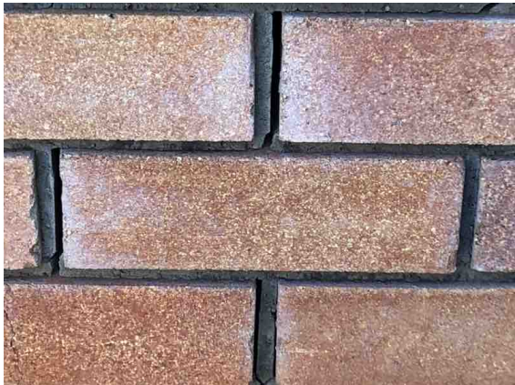
Stepped cracking
