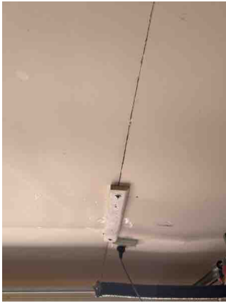
Sagging and cracked ceiling
