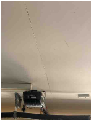
Sagging and cracked ceiling
