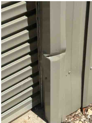
Damaged cladding
