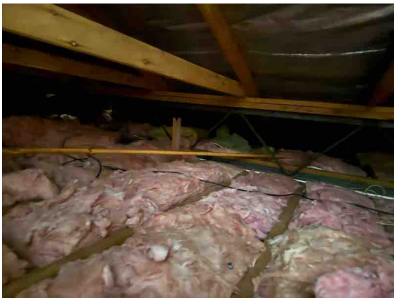
Insulation in the roof void area.
