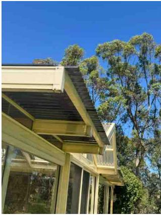
The missing gutter. The end of the sheeting needs extra screws installed.
