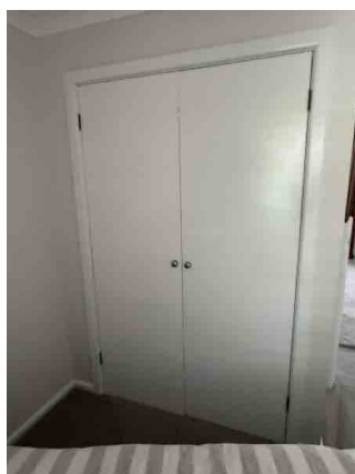
The bottom of the doors needs to be eased on the cupboard.
