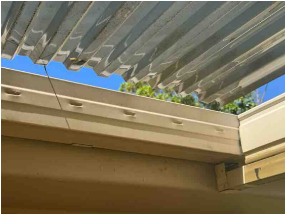
The missing roof flashing and loose sheeting.
