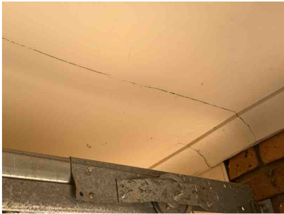
Sagging and cracked ceiling.
