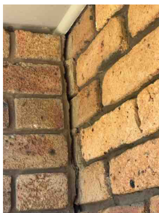
Wall cracking in the brick pier.
