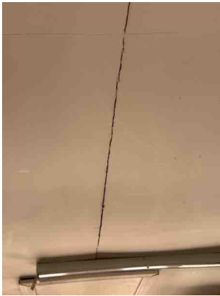
Sagging and cracked ceiling
