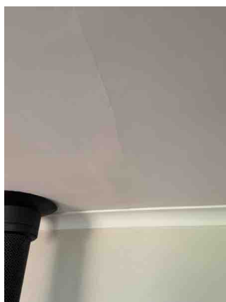
Ceiling cracking
