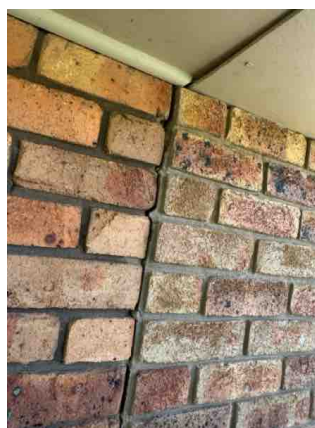
Wall cracking and movement.
