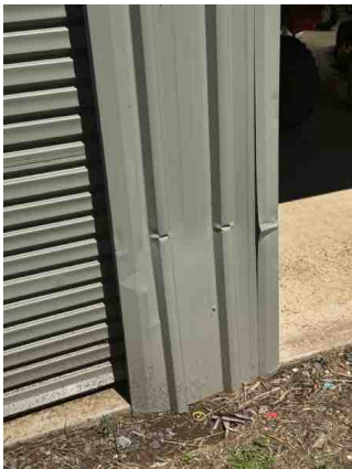
Damaged cladding
