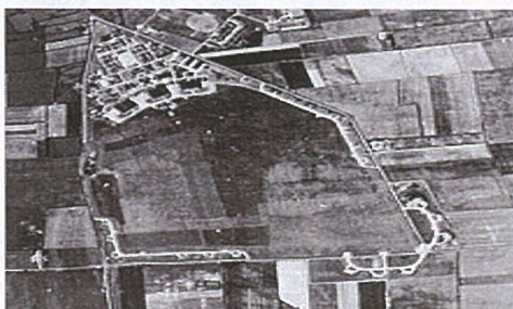
Figure 5: Aerial photograph of RAF Kirton in Lindsey, showing the technical site with three C-Type hangars to the top (north), 27 July 1948. (Americanairmuseum.com)
