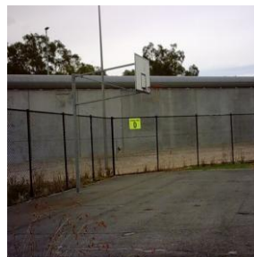
Image 17: Concrete walls and basketball court
