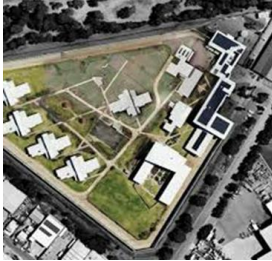
Image 1: Aerial view of AYTC Image taken from google images
