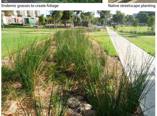
Bio stormwater bio swale
