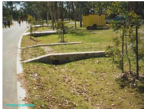
Photo*: Grassed swale with adjacent driveways, Cairlea, Brisbane Queensland.
