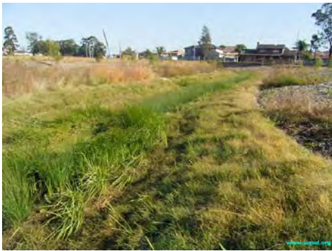
Photo*: Vegetated swale, Fairfield New South Wales
