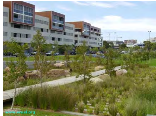
Photo*: Bioretention basin, Victoria Park, Sydney.
