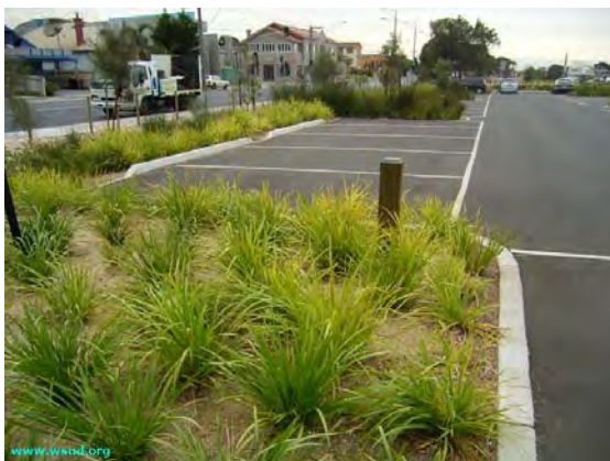
Photo*: Example of rain garden (bioretention basin) adjacent to car parking bay at Beachside Car park (Melbourne), Victoria.
