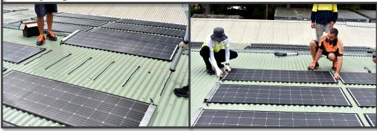
Silicone is applied using a Cordless Caulking Gun. 5-8 mm bead is applied at equal distance (as per installation manual). 2 installers are used to ensure module is installed square. NOTE Avoid screw lines when placing panels.
