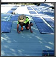
Set out array allowing for efficient application of silicone and ensuring the array is square.
