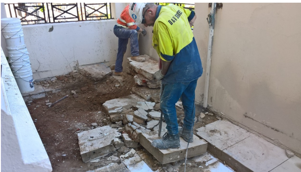
Image 2 – Concrete slab section further broken down to enable removal by hand
