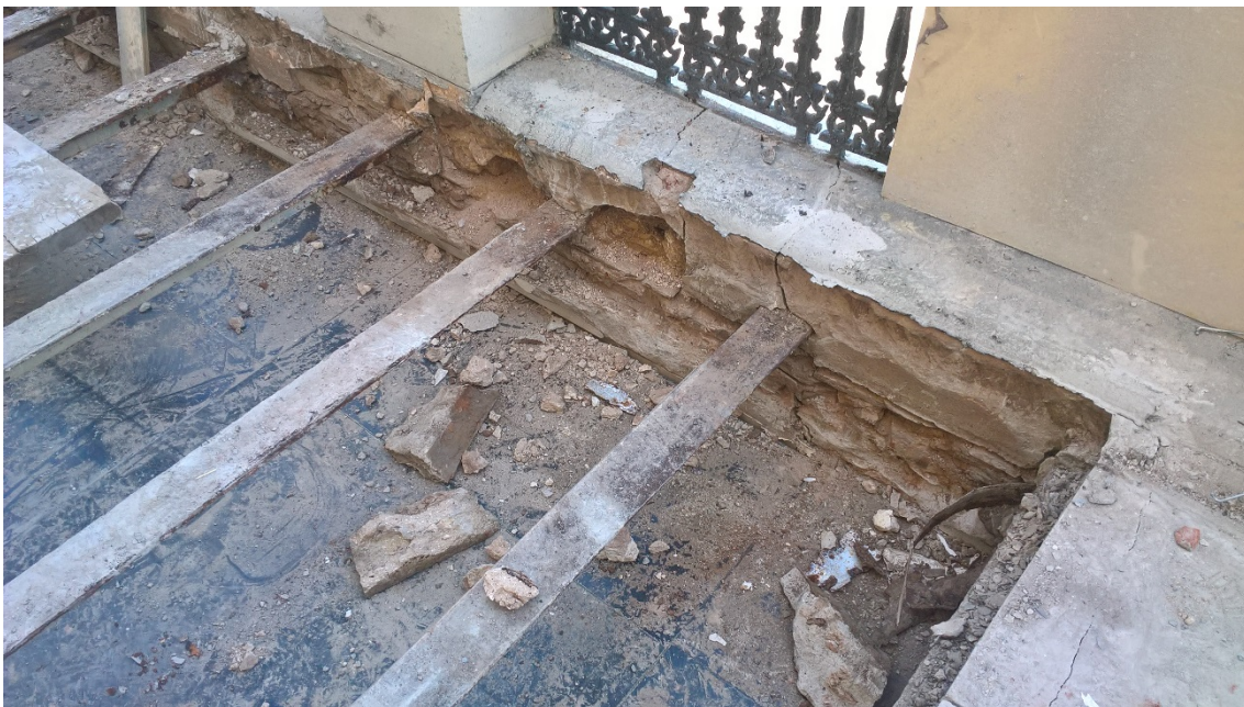
Image 6 – Corroded steelwork of the Town Hall balcony and clay instead of stone construction exposed.
