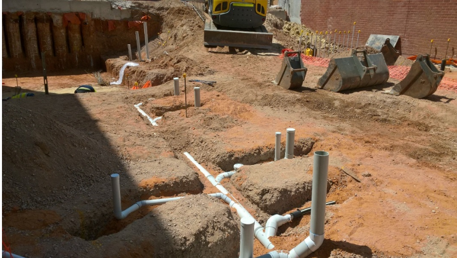
Image 11 – New building ground floor plumbing pipework installed
