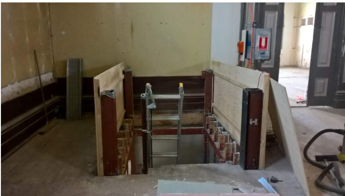
Image 15 – The lift shaft structure partially removed
