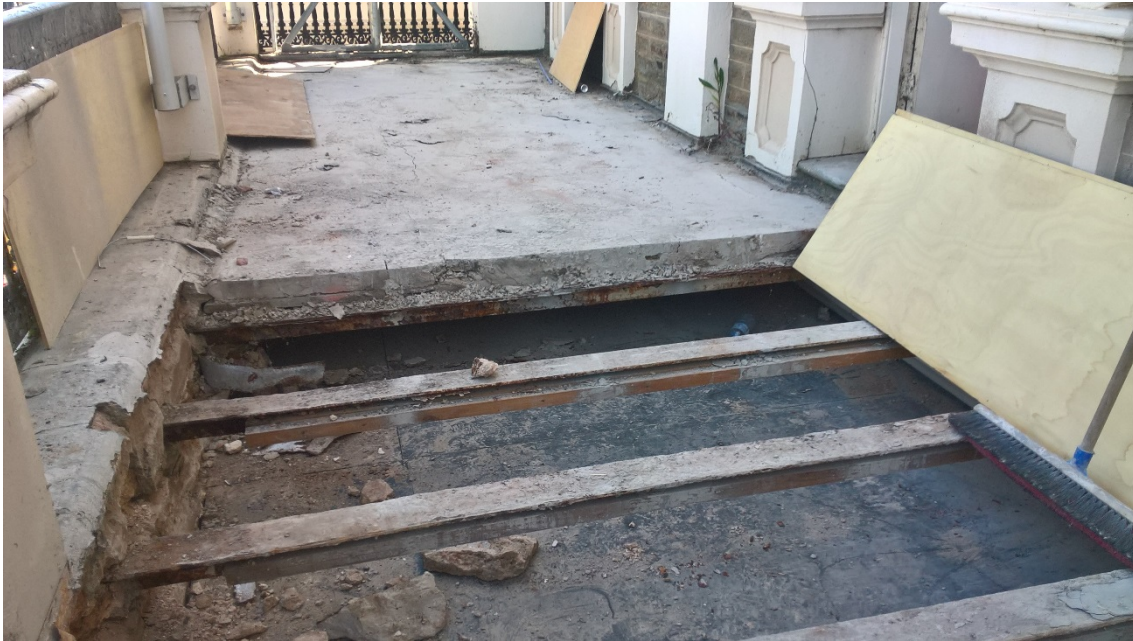
Image 5 – The Town Hall balcony partly demolished exposing the steel structure
