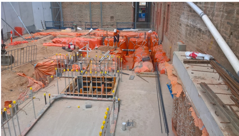
Image 13- Ground floor footings partially poured with concrete reinforcing installed
