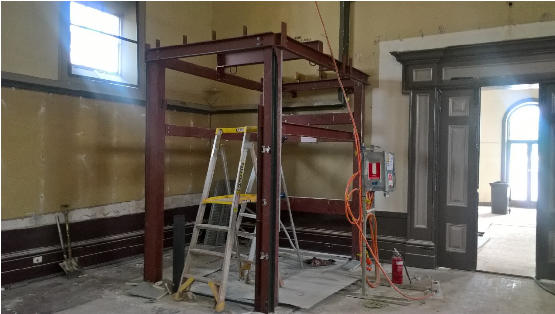
Image 14 – The lift shaft cladding removed
