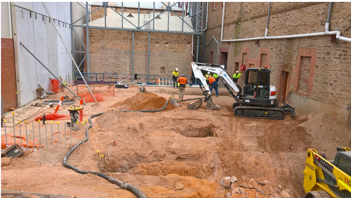
Image 10 – New building ground floor footing excavation in progress
