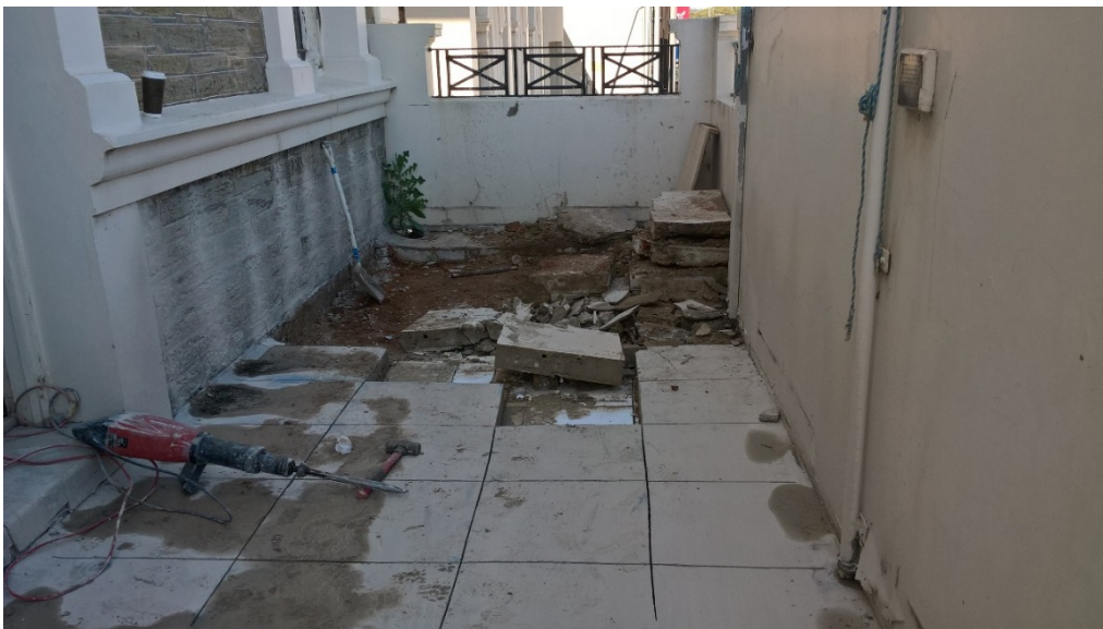
Image 1 – Existing concrete slab cut into sections ready for removal.
