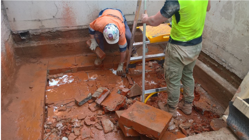
Image 3 – Brick work and soil discovered under the balcony concrete slab
