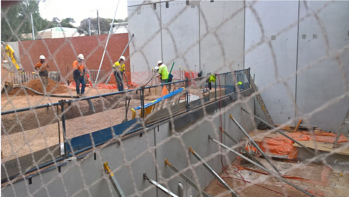
Image 9 – The precast concrete retaining wall of the basement now backfilled.
