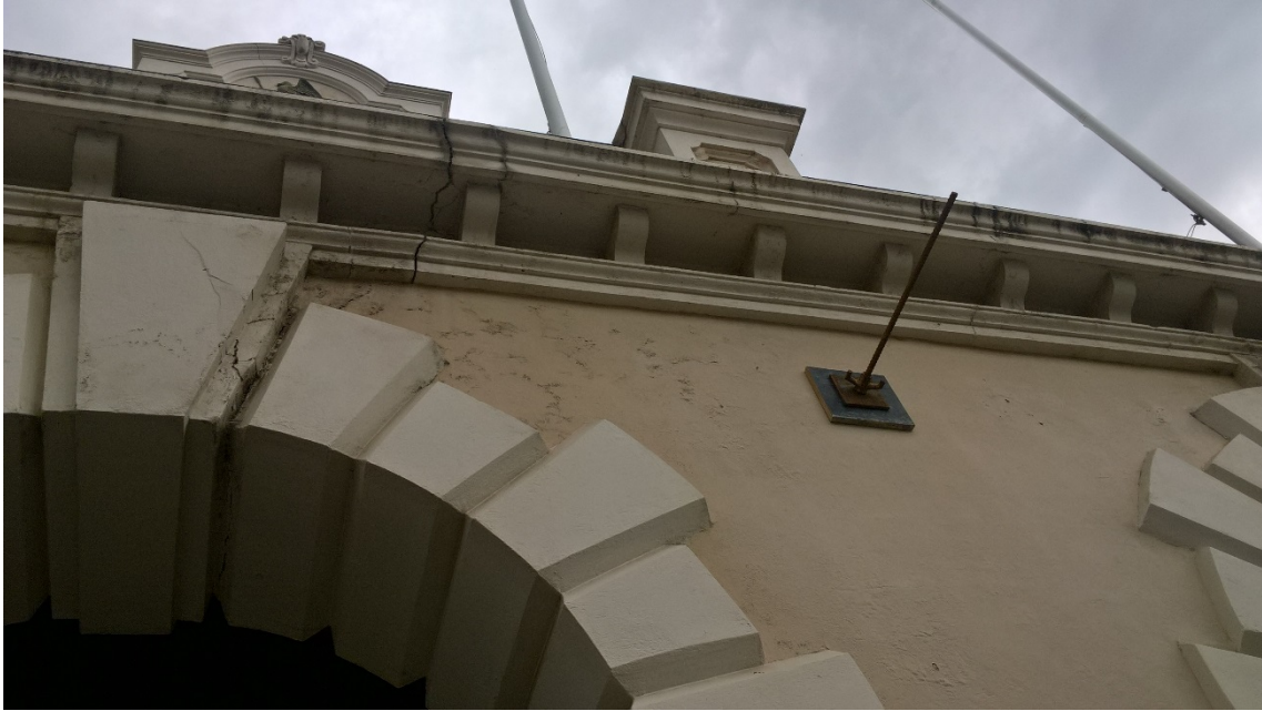
Image 7 – The existing crack in the Town Hall arch
