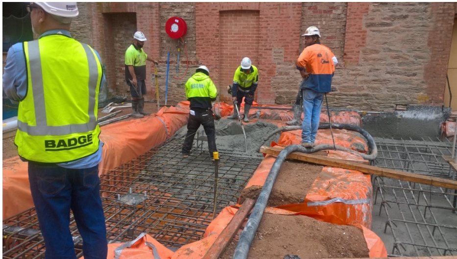
Image 12 – New building ground floor footings being poured
