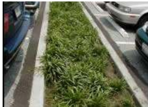
Fig 9: Bio-retention Cell incorporated into a car park
