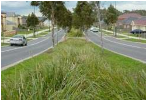
Fig 4: Typical Planted Bio-retention Swale. (University of Nevada)
