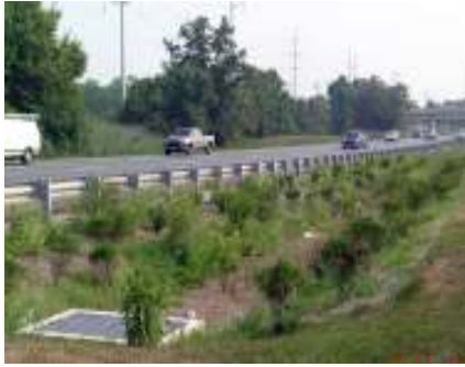
Fig 6: Typical Roadside Bio-retention Basin
