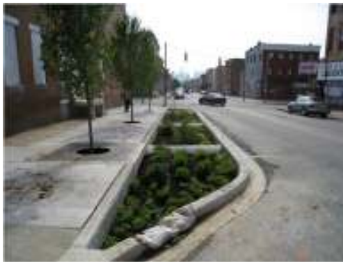
Fig 8: Bio-retention Cell incorporated into a Streetscape environment
