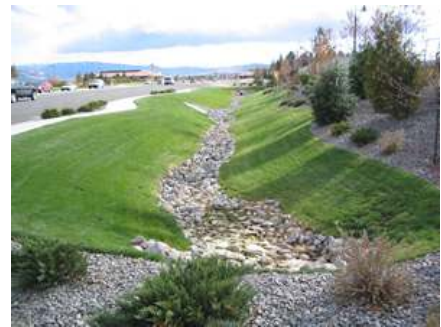
Fig 5: Bio-retention Swale with Scour protection. (Melbourne Water)
