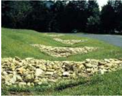
Fig 1: Grassed Swale with Check Dams
