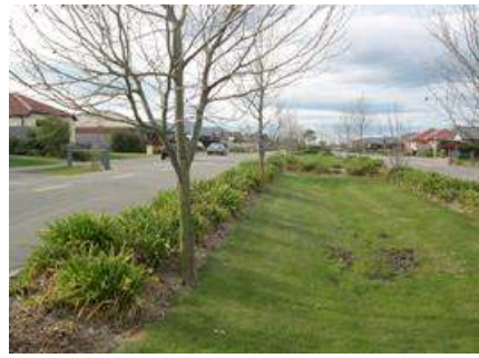
Fig 2: Roadside Grassed Swale
