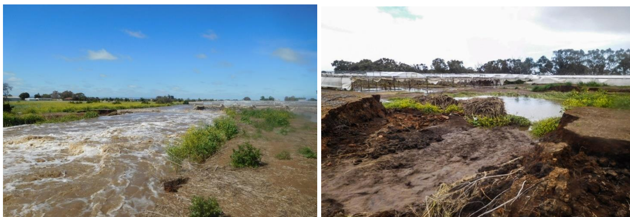
Figure 3.1 Levee breach during 2016 flood event
