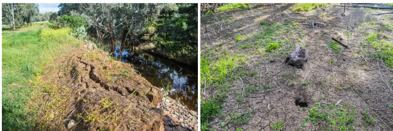
Figure 3.2 Example of levees in need of immediate repair
