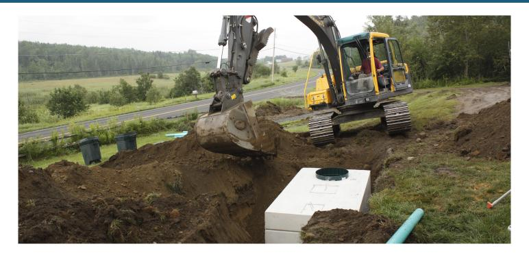
Many properties in Gawler's rural areas such as Kudla and Hillier are not connected to a sewer system. Therefore these properties require wastewater systems to dispose of liquid waste from the kitchen, laundry, bathroom & toilet.
