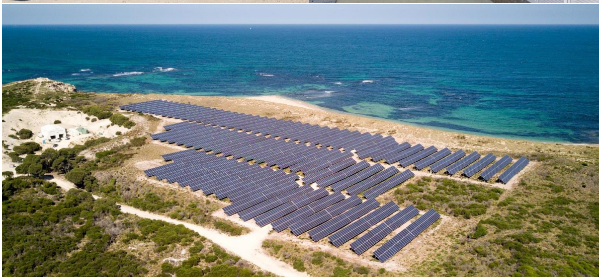
Garden Island Microgrid Project
