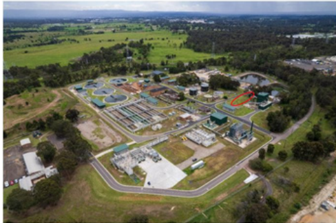
Aerial view of Riverstone WRRF (approximate carboniser location in red)
