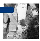
When the first course is in place, backfill behind the blocks with a minimum 300mm wide 10-20mm blue metal drainage aggregate to a level slightly lower than the block height. Lay in the second block course then backfill immediately behind the wall with the drainage aggregate.
