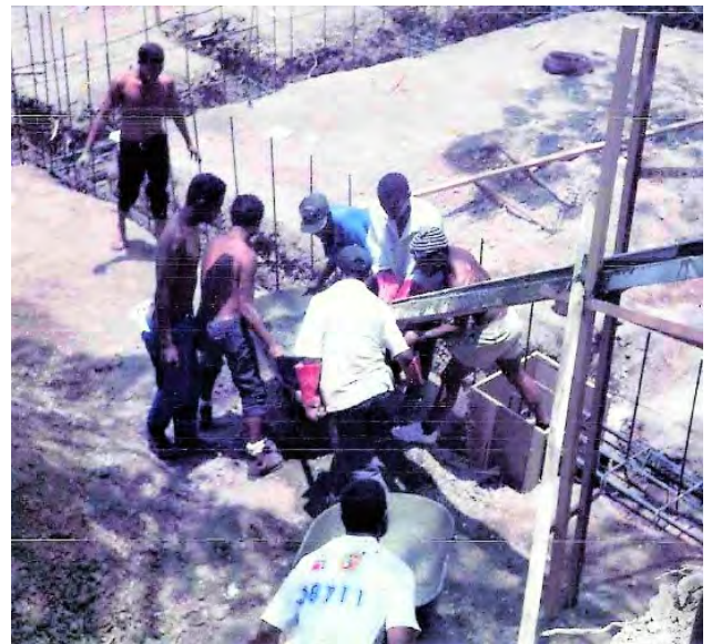
16: Students & Staff pouring concrete for 1995 Building
