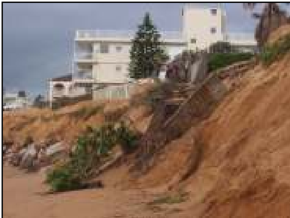
Figure 6g: Erosion along Collaroy/Narrabeen Beach on 18 th June 2007 (Courtesy Department Environment & Climate Change)
