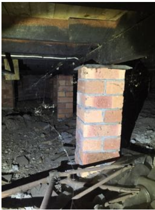
Slightly rotating piers middle area
