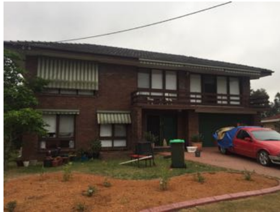
2 Gretel Crescent Booragul (Southern Elevation)
