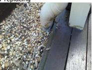
Flashings Dented and will need repair to restore appearance
