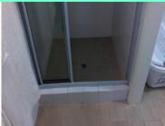
Door Sliding door guides are broken or missing and need repair or replacing to ensure correct operation/function
