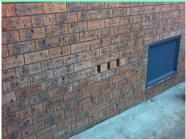
Bricks fretting Minor fretting was noted in some areas, if further deterioration is noted replacement of
