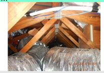
Framing Timber truss framing is OK
