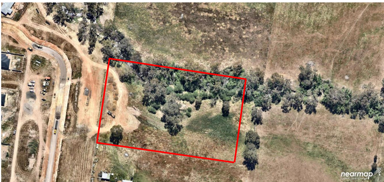
Figure 4: Site Aerial Photo. Image Source: Nearmap
