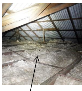
Insulation obscured timbers
