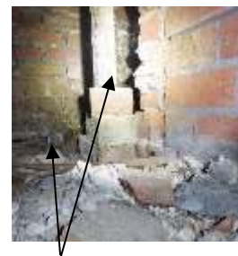
Remove timber from ground
