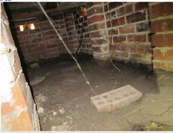
Drainage Inadequate, I recommend the subfloor drainage is improved, improving the site drainage may
