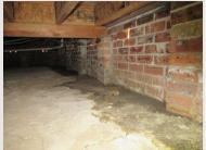
Drainage Inadequate, I recommend the subfloor drainage is improved, improving the site drainage may
