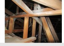
Framing Timber Truss framing is OK
