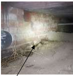
Remove timber from ground
